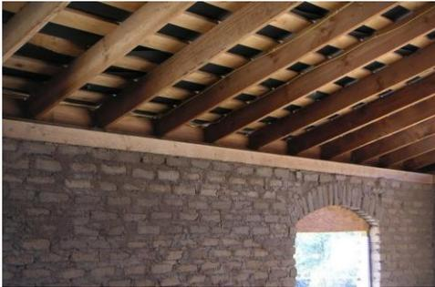
Almost all passive solar systems work in conjunction with **thermal mass**, or materials with a high capacity for absorbing and storing heat (e.g., brick, concrete masonry, concrete slab, tile, adobe, water). Thermal mass can be incorporated into a building design as floors, interior walls, fireplaces, or bancos. The sun does not need to hit these surfaces directly to store the heat, nor do these surfaces necessarily need to be a dark color. The thermal storage
